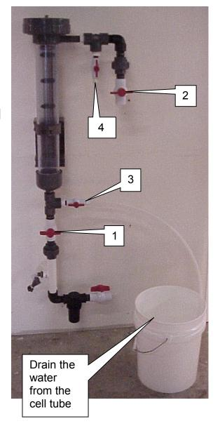
Connect the acid wash tank and pump to the acid wash valves [3] and [4] as shown in the photo on the right.
